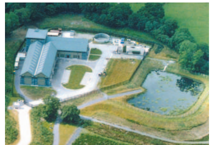
Example of remote pumping station.
